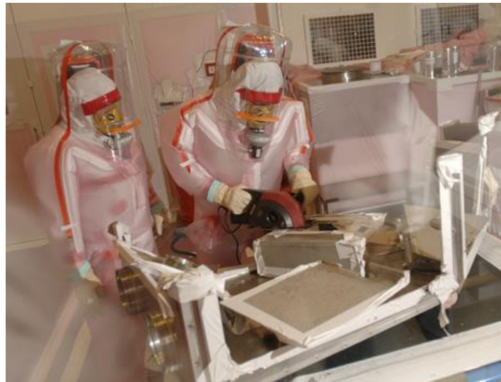
Dismantling mixed oxide production facility
