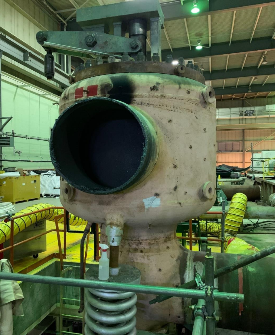
Combined Intercept Valves & steam lines to be removed up to Rx Building
