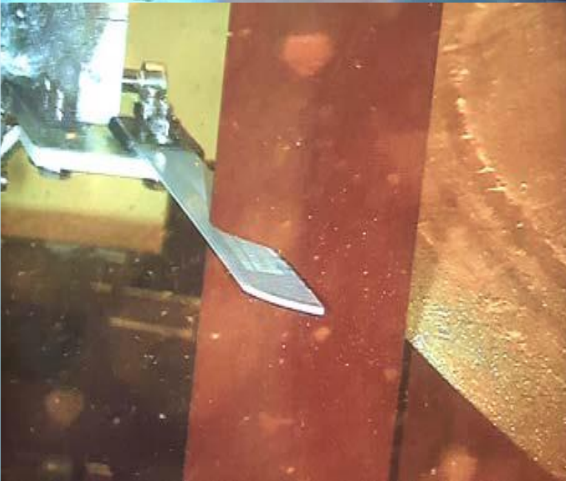
Underwater camera photos of cutting lifting lug(s) off the Steam Separator
