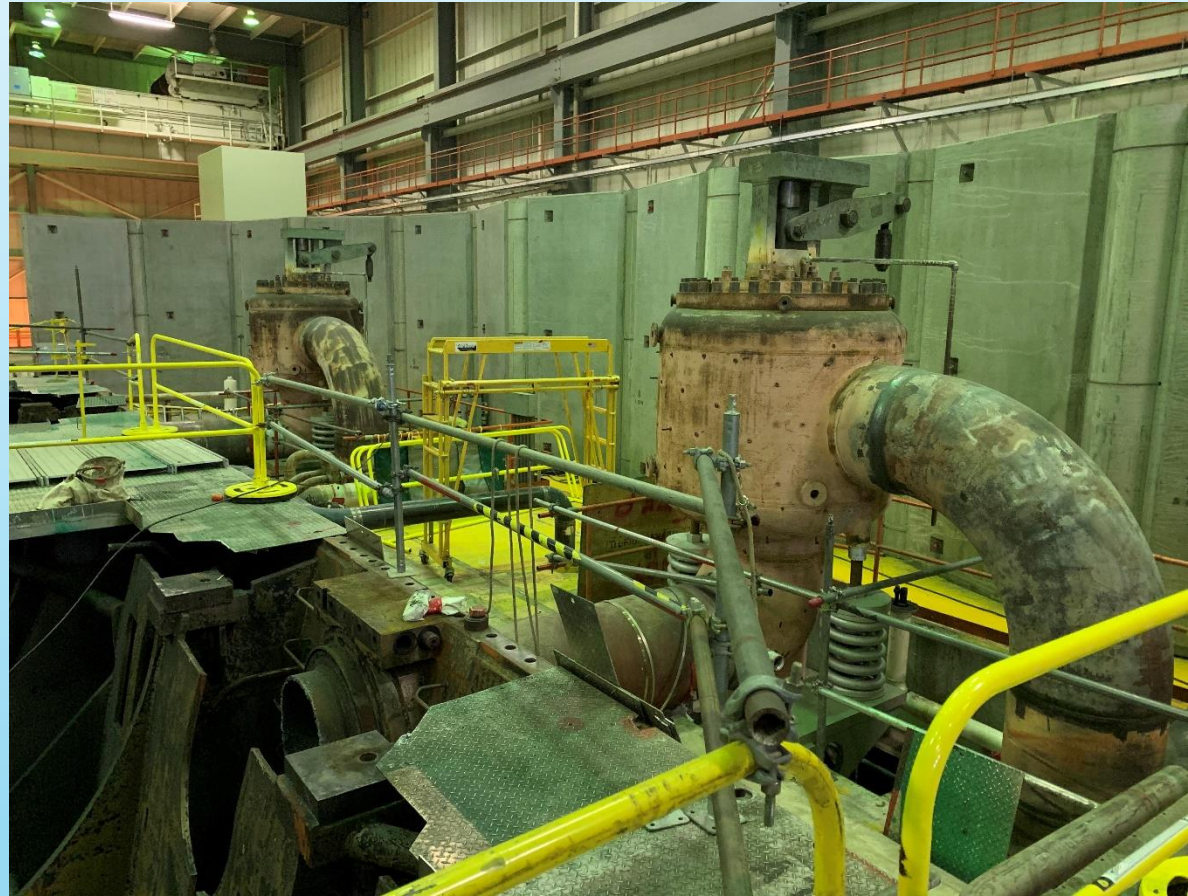
Turbine to Condenser opening with CIVs (which are being removed) in background
