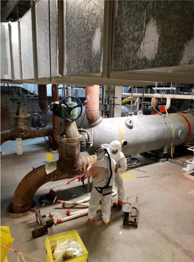
Workers prep to cut Feedwater system piping/valve for removal.
