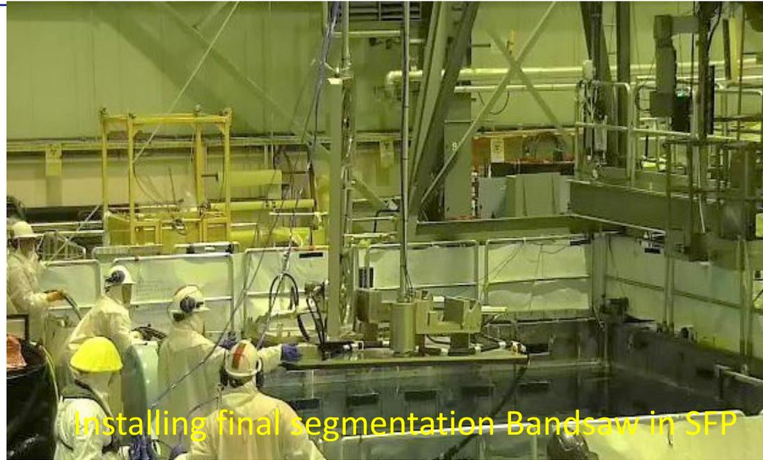
Installing final segmentation Bandsaw in SFP
