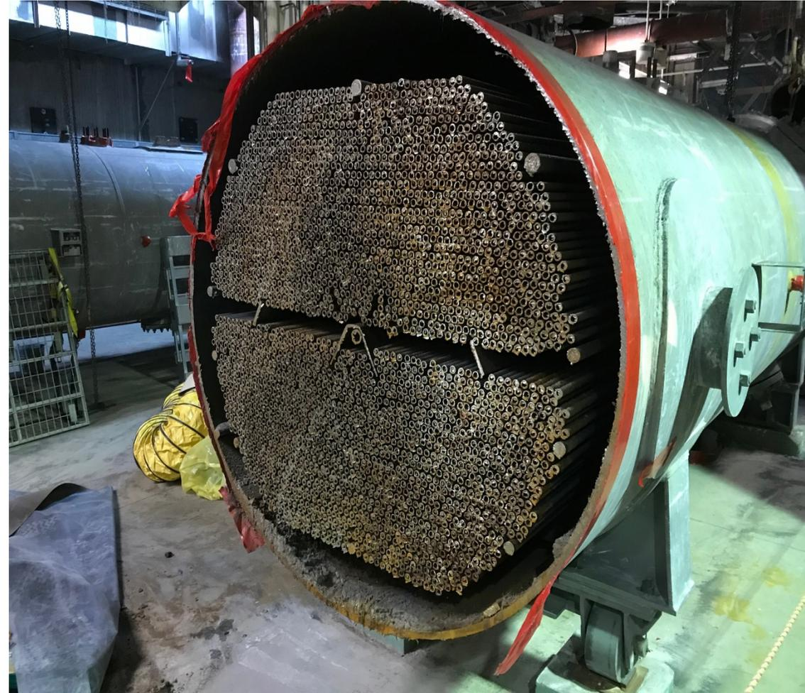
Diamond wire saws used to reduce large components into manageable sized pieces. (1/2 of a Feedwater Heater shown)
